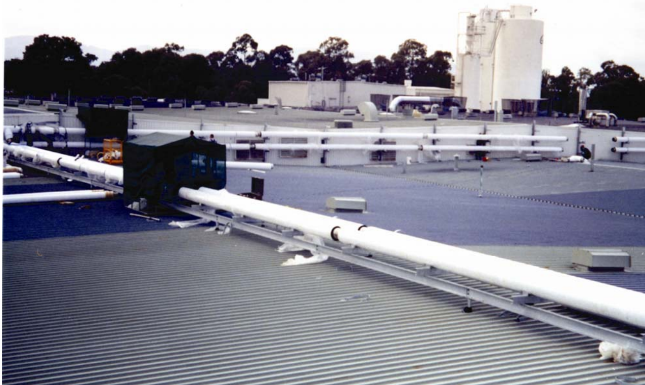
■ Cadbury Australia - Air-conditioning installation
