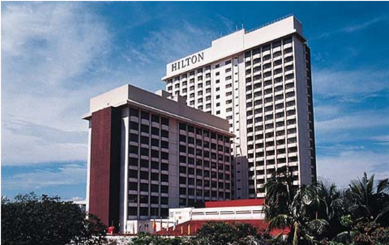
■ Petaling Jaya Hilton Hotel - Air- conditioning retrofit - chilled water service
